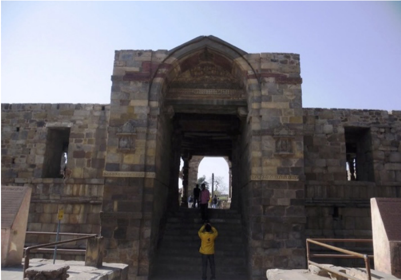
Fig. 2. Qutb Mosque, entrance portal.
