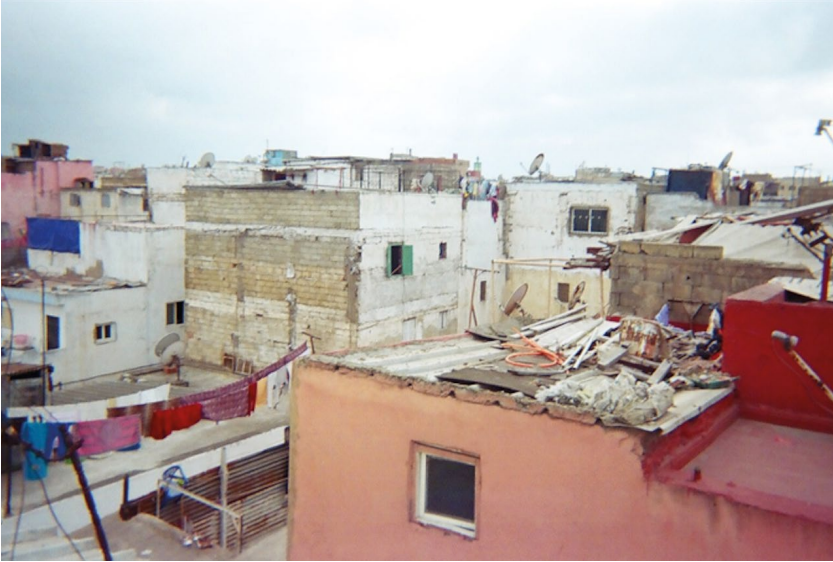
Figure 2: Rooftop view of the appropriated grid.
