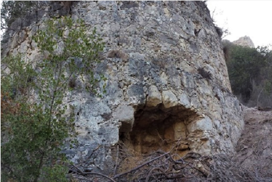
Fig. 19: Undermining of the administrative building (a) and the south-western tower (b) (© Adrian Boas and Rabei Khamisy).
